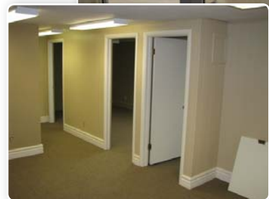
New Carpeting, sheetrock and painting in June.
