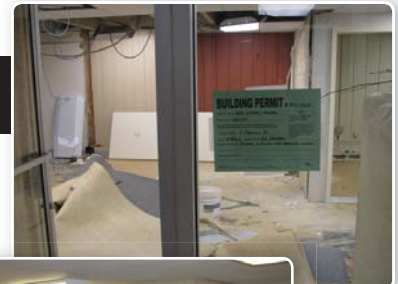
Deconstruction of the rooms in May.
